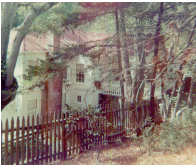
877 Madison Street, the house in the hole.
