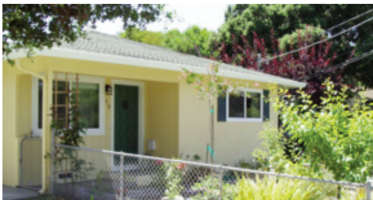
Before and after of Casanova house.
