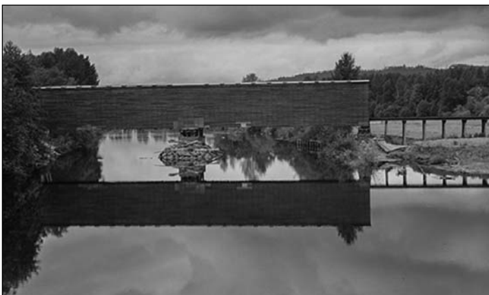
Covered RR Bridge with partial view of Matt & Sophia Forstrom's former "bridge site."
