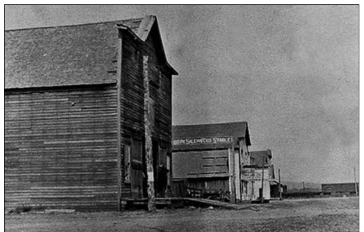
Above: Helsing Junction, buildings deteriorating, ca. 1940s-50s.
