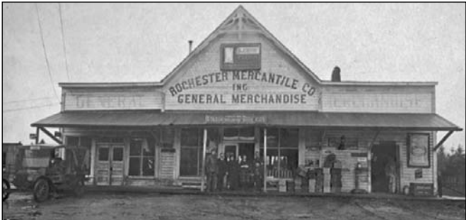
Above: Three views of the Post Office and the Rochester Mercantile on Highway 12 (183rd Avenue).
