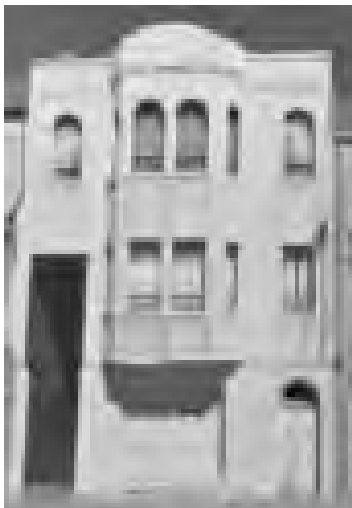
The 2-flat building at 1838-1840 Greenwich, still owned by Ray Martelli as of 2022.
