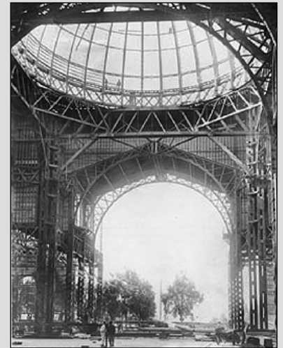
Dome under construction, 1914.
